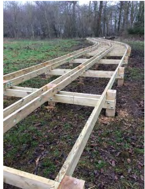
Fig 11 - Kingston Lacy, boardwalk subframe under construction
