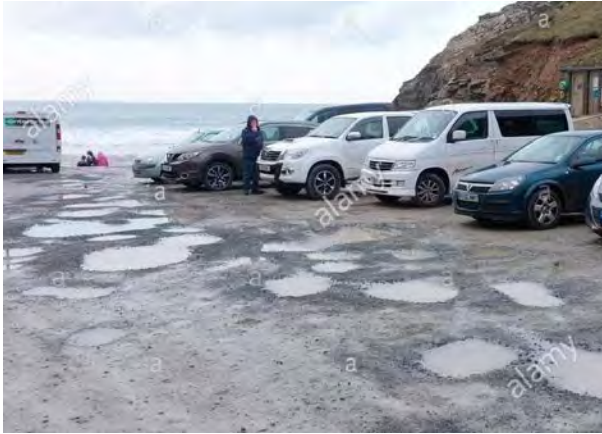
Fig 17- simple stone car park with excessive deformation
