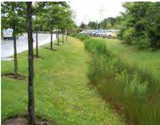
Fig 25 - swale to perimeter of construction
