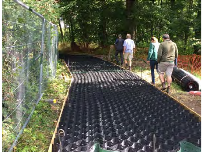
Fig 13 - ongoing installation to BS 5837 at Kingston Lacy; note timber edge boards and heras fencing
