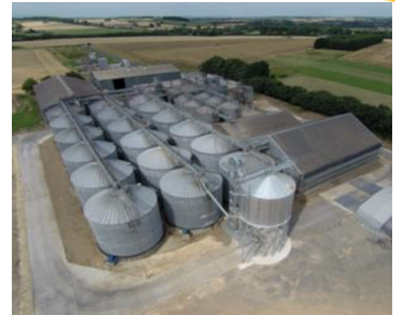
Grain storage 1,000,000 mt of grain storage
